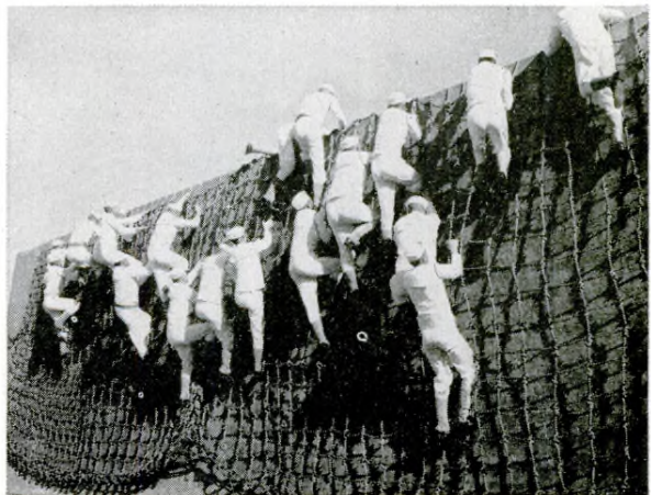
FIGURE 5.—Obstacle course—cargo nets over the side.
